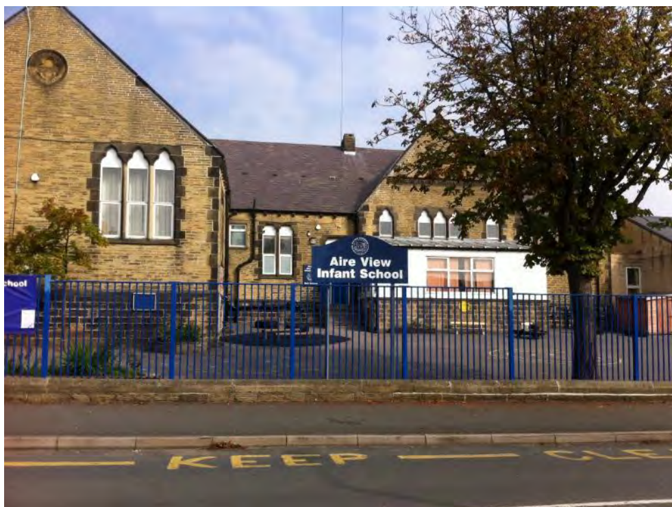
Aire View School, Silsden
