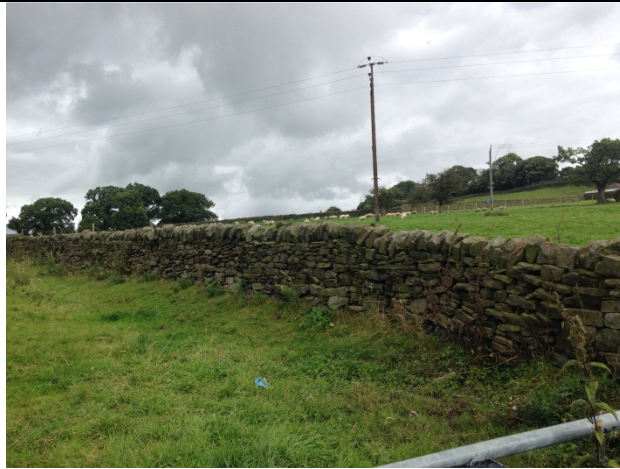
DRYSTONE WALL ADEJECENT TO FOOTPATH 44
