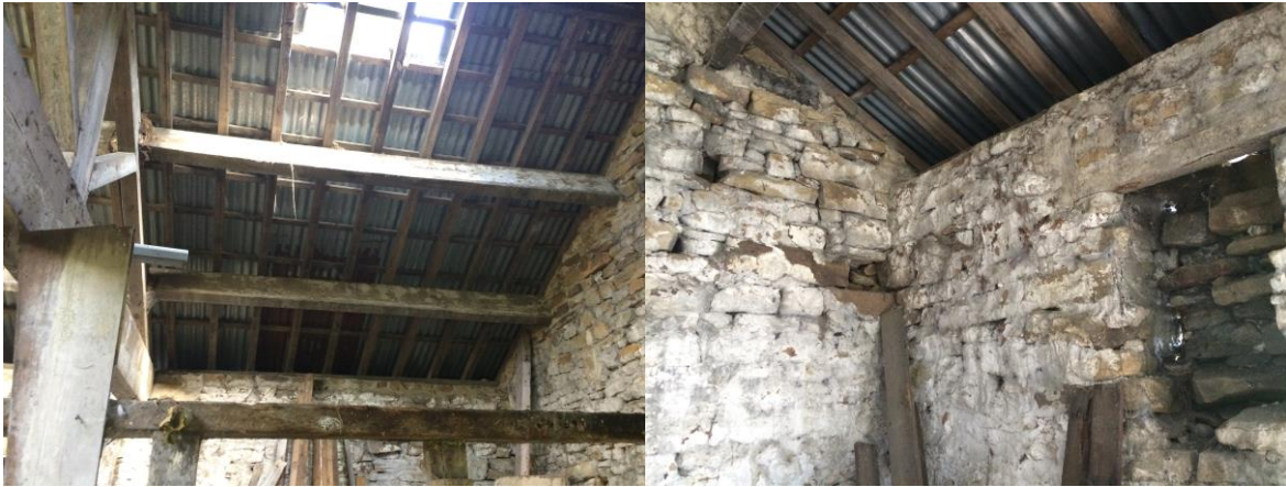
Figure 9 Interior of the barn
